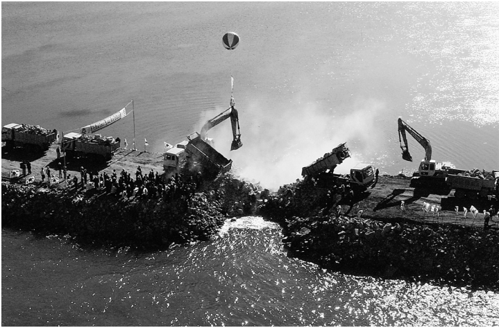
Figure 11. Land reclamation work for the development of Songdo, showing early stages of shoreline infill. Courtesy of Incheon Metropolitan City.
